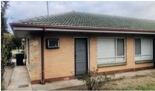
Unit 1, 362 Hampstead Rd, Clearview
