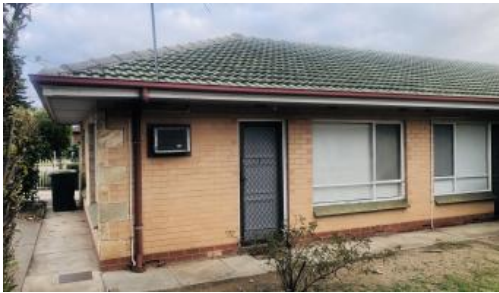
Unit 1, 362 Hampstead Rd, Clearview
