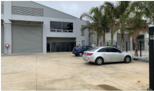
Unit 2/ 43 Ellemsea Cct, Lonsdale
