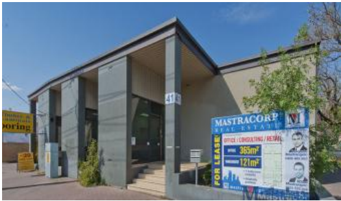
41A Goodwood Road, Wayville
